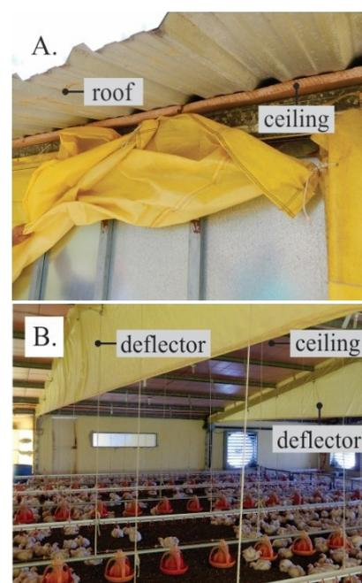
**Figure 1.** Details of flexible closing, roof and ceiling (A) and air deflectors and ceiling (B)
